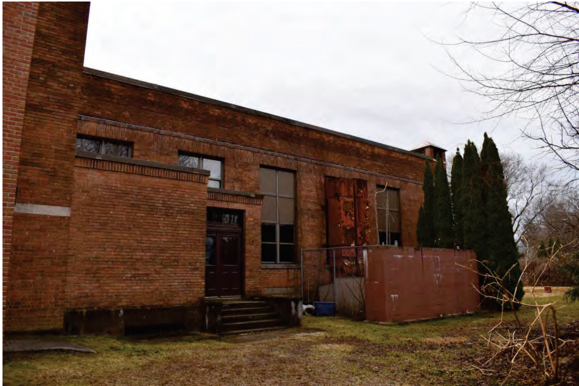
Photo 4: Buried utilities and equipment are located on the northern side of the school building. View to the southwest.
