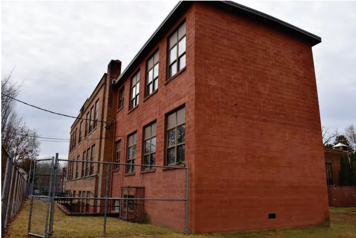
Photo 5: The northern side of the building is constructed of cinderblock, and painted red. View to the south.
